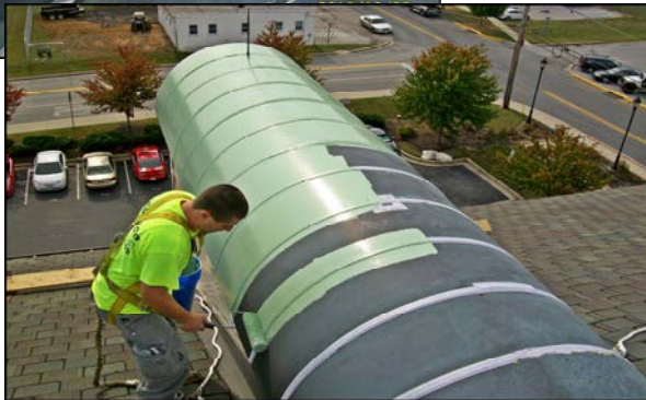
WESTMINSTER COURTHOUSE DORMER / ROOF WATERPROOFING TRUCO SYSTEM 10 YEAR WARRANTY CUSTOM COLOR
