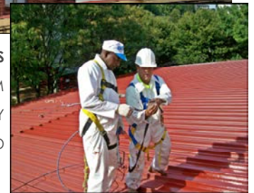
QUALITY CONTROL INSPECTING MIL THICKNESS
