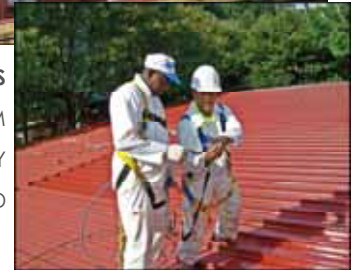
QUALITY CONTROL INSPECTING MIL THICKNESS
