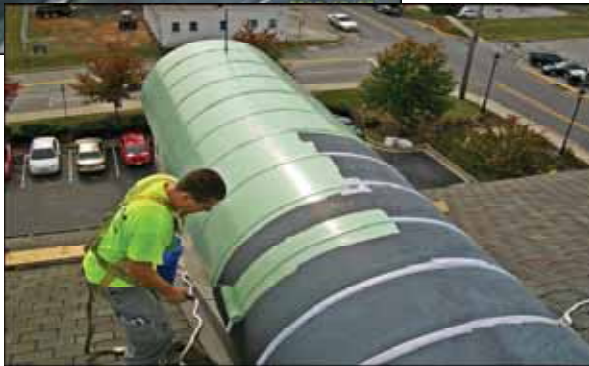
DORMER / ROOF WATERPROOFING TRUCO SYSTEM 10 YEAR WARRANTY CUSTOM COLOR
