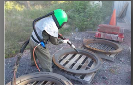
Manhole Covers Vapor Blasting
