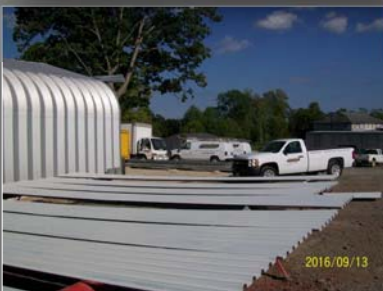
Ceiling Panels Epoxy Primer Urethane Finish
